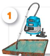
• Drain pan then use a wet vacuum to remove any water or loose deposits from the surface.
